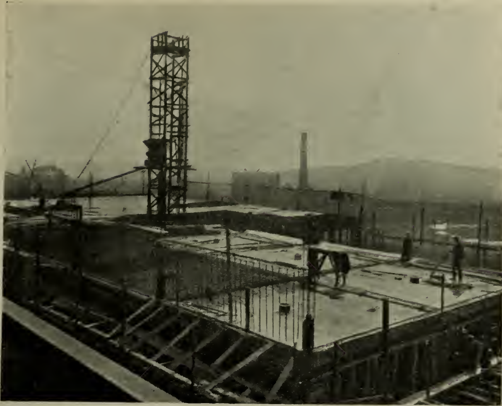
PROVAN GASWORKS : Part of Revivifying Floor.
